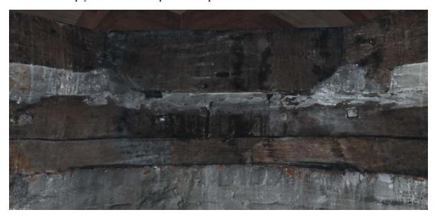
The mortise where the sprattle beam (which supported the vertical shaft) was removed is clearly visible. Site investigations suggest that the corners of the rectangular cap frame, including the shear beams (which supported the fantail) were cut away. Any surviving physical evidence of the toothed rack which would have run around the outside of the curb is impossible to examine because the exterior brickwork is laid closely against the outside face of the curb.
